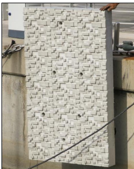
a) Installation of an eco-seawall
