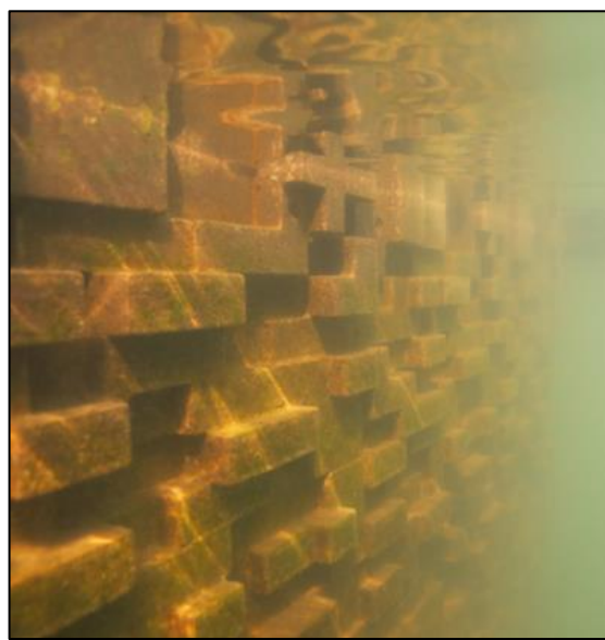
b) Eco seawall submerged under high tide
