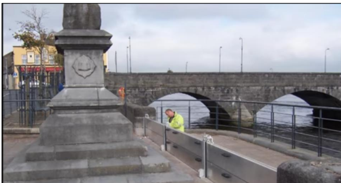
Plate 4.6 Demountable Flood Barriers at Clancy Strand, Limerick (Source: www.floodgateireland.com )
